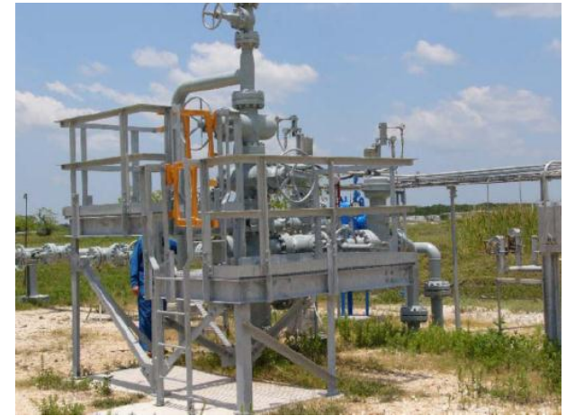
Outlet valve of a hydrogen cavern
